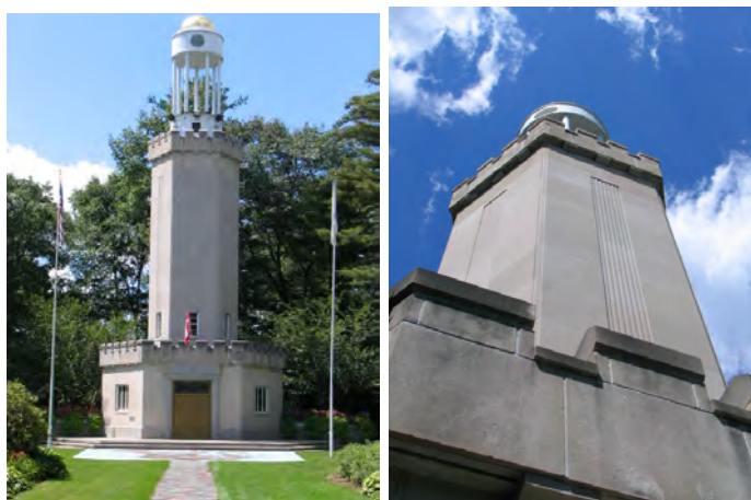
Figure 6.3: The Carillon Tower at Stanley Park in Westfield, MA; front view and view from base.
